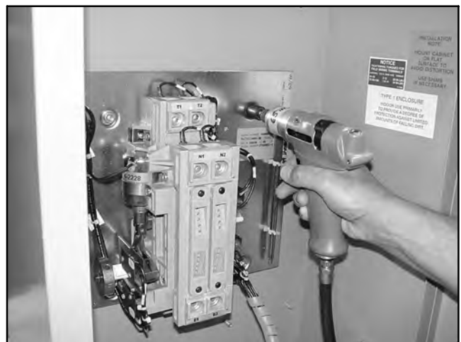
Figure 6-6 Installing the Power Panel
