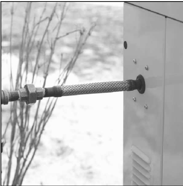
Figure 3 Fuel Connection
