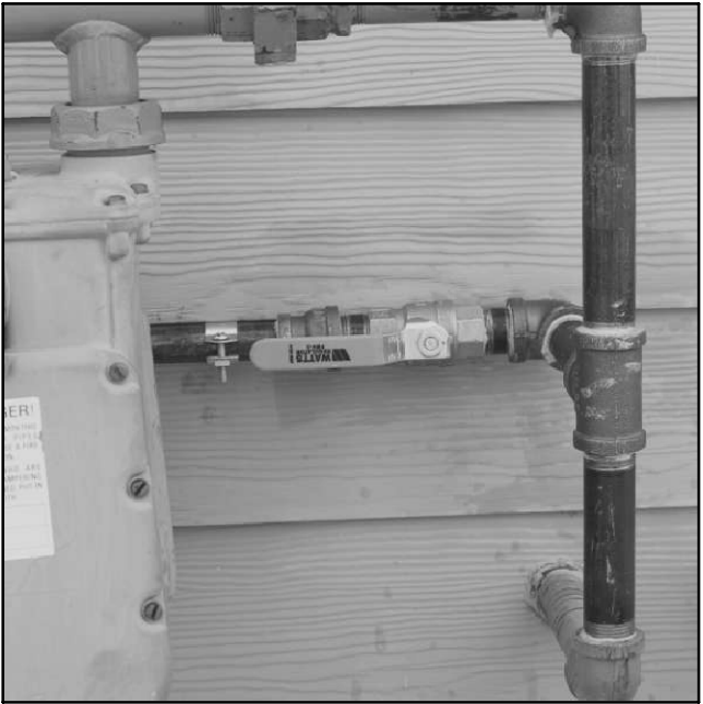
Figure 1 Manual Fuel Valve (provided by fuel supplier)
