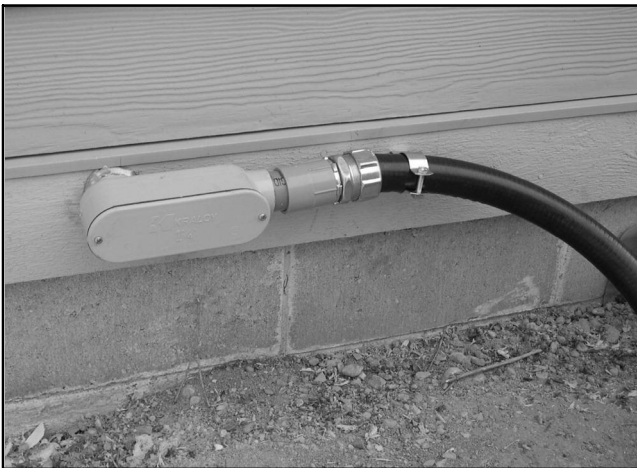
Figure 6 Wiring Kit Plastic Elbow Mounted to Wall
