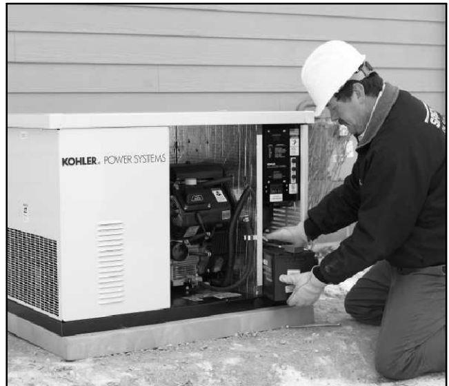
Figure 14 Battery Installation
