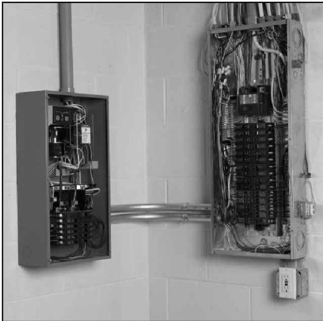
Figure 13 ATS and Main Distribution Panel
