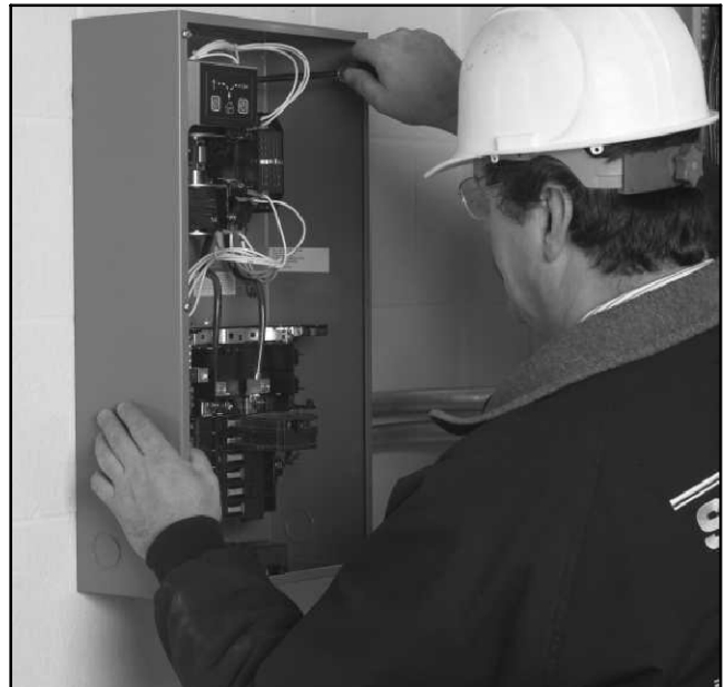
Figure 4 Mounting the Transfer Switch
