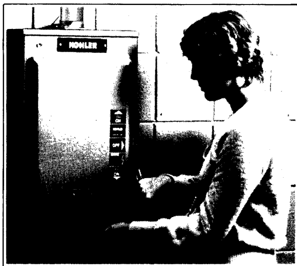
Figure 1-8. 200/100 Amp. Transfer Switch
