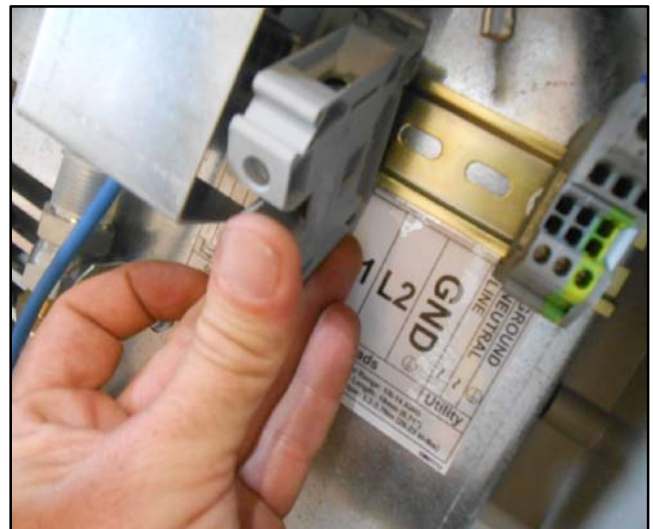
Figure 8 Installing the New Terminal Block
