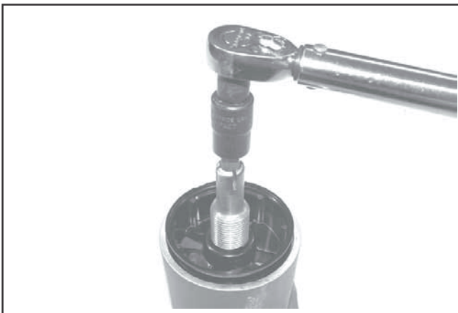
Figure 10-68. Torquing Nipple.
