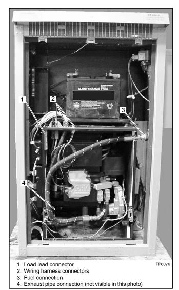
Figure 6-1 Generator Set Installed in the cabinet
