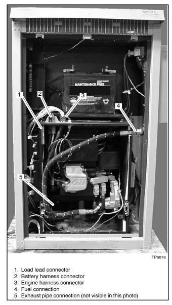
Figure 2-1 Generator Set Installed in the Enclosure (front panel and door removed)
