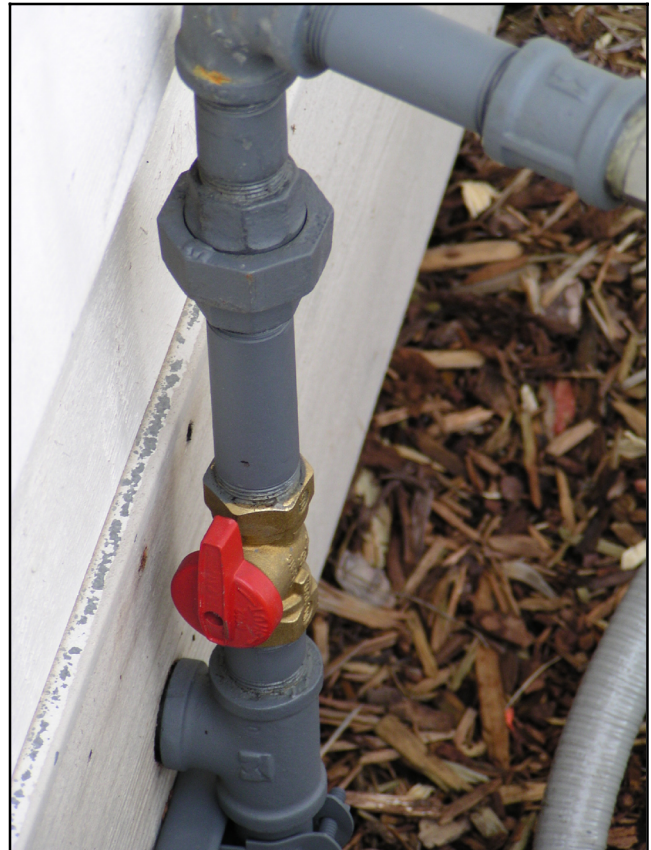
Figure 3-8 Manual Fuel Shut-Off Valve (outdoor installation shown)
