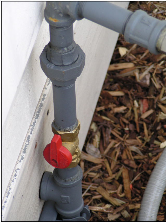
Figure 2-8 Manual Fuel Shutoff Valve (outdoor installation shown)
