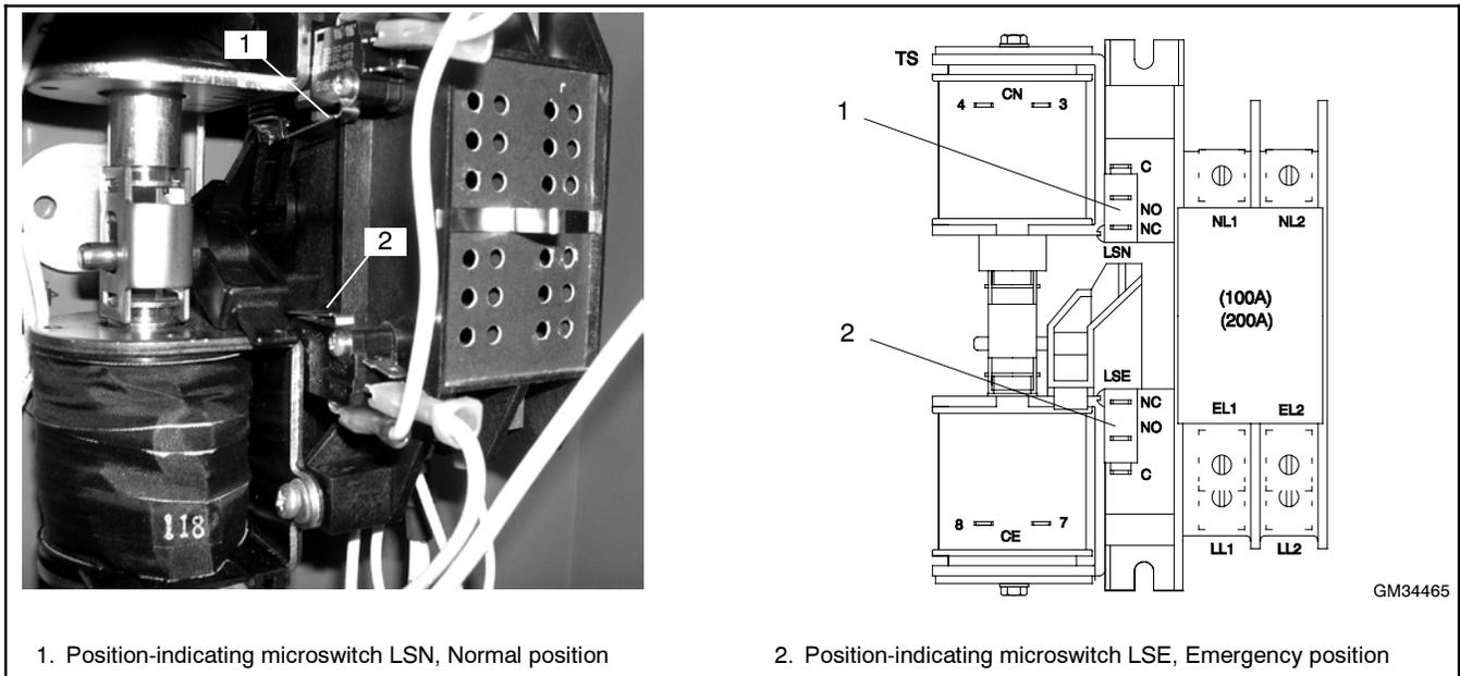
**Figure 5-13** Position-Indicating Microswitches, 100/200-Amp Models
