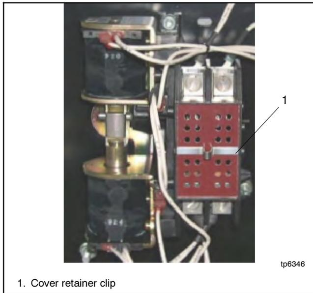
**Figure 3-3** Typical Arc Chute Cover, 100/200 Amp Models
