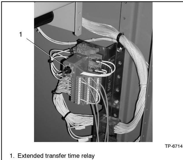
**Figure 1-5** Extended Transfer Time Relay
