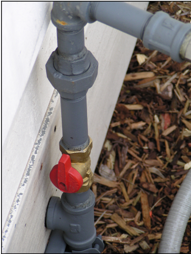
Figure 3-7 Manual Fuel Shut-Off Valve (outdoor installation shown)
