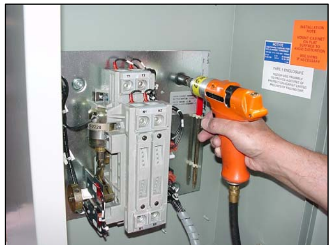
Figure 7-7 Installing the Contactor
