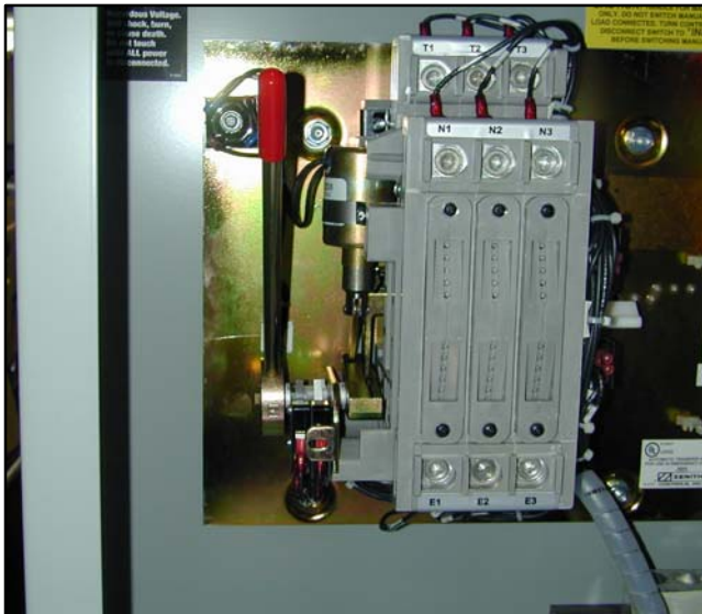
Figure 7-39 Manual Operation Handle Inserted
