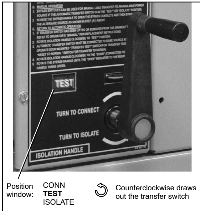
Figure 7-15 Isolation Handle Turned to TEST
