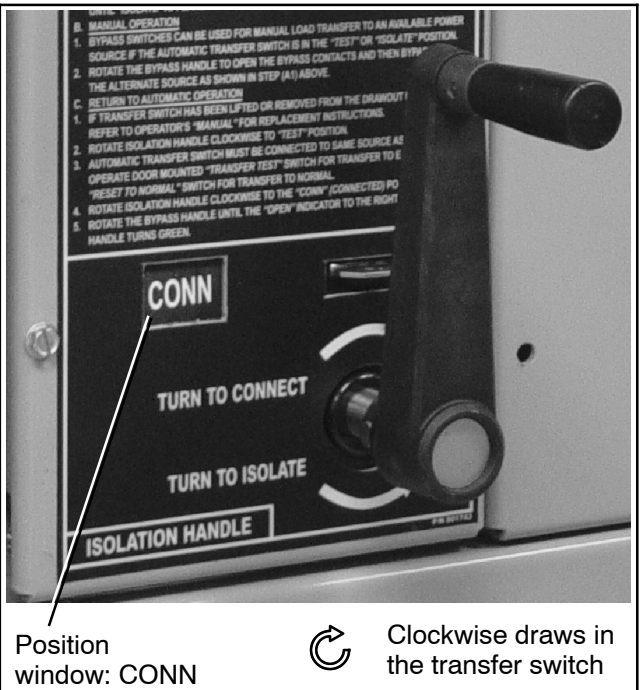
Figure 7-24 Isolation Handle Turned to CONN
