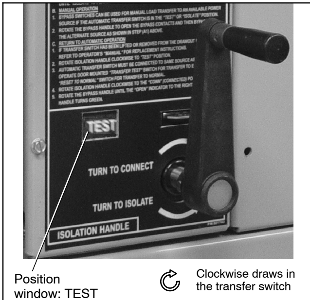
Figure 7-22 Isolation Handle Turned to TEST
