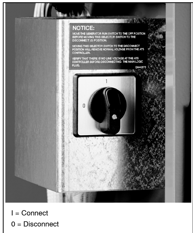
Figure 4-6 Controller Disconnect Switch
