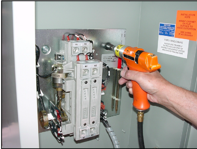
Figure 7-6 Installing the Power Panel
