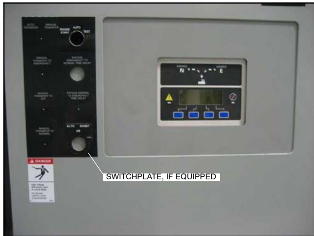
Figure 31 Before Decal Installation
