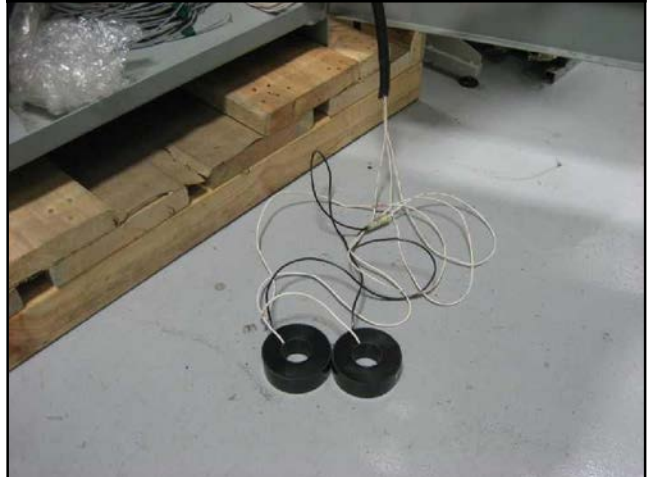
Figure 6 Current Transformers (CTs)
