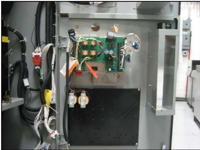
Figure 13 Transformers and Terminal Block Removed from Lower Panel but Not Disconnected
