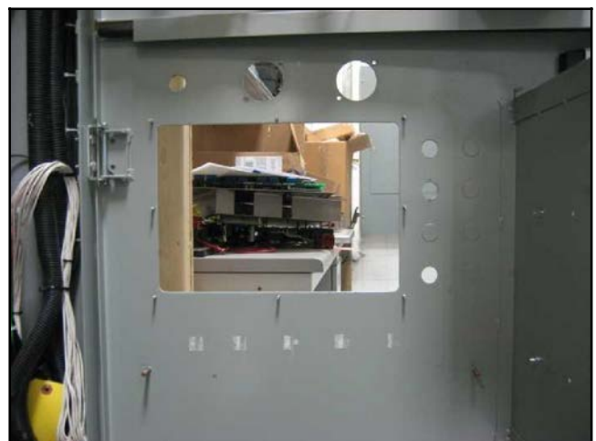
Figure 21 Controller and Lower Panel Removed
