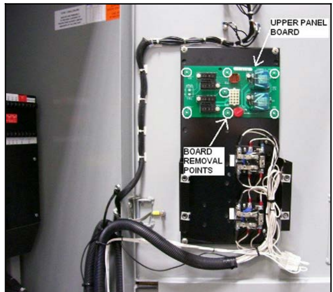
Figure 49 Remove the Upper Panel Circuit Board
