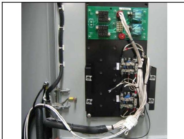
Figure 45 P8 has been disconnected from the upper board and connected to conversion kit harness GM69403.
