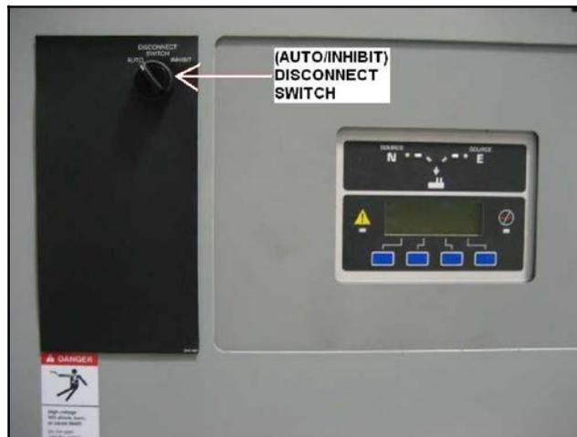
**Figure 33** Disconnect Switch Re-Installed
