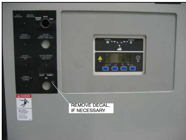
**Figure 31** Remove Auto/Inhibit Switch Decal (if necessary)
