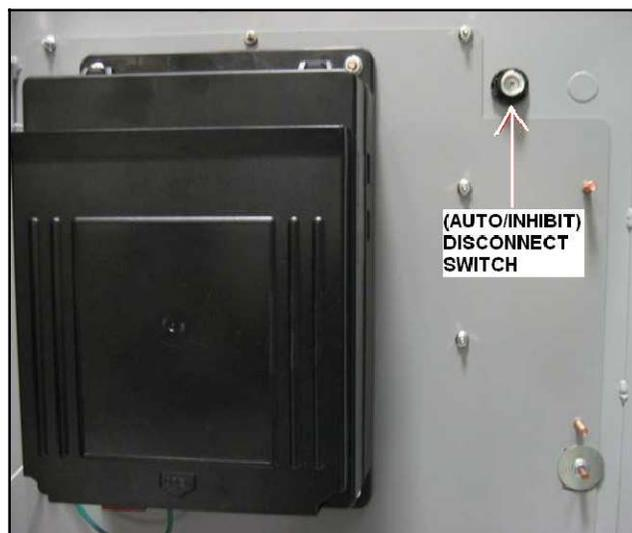
**Figure 34** Disconnect Switch (inside door)
