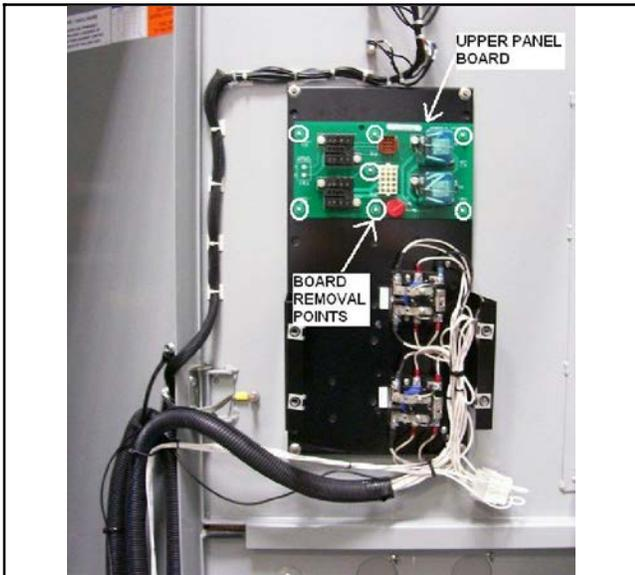
**Figure 50** Remove the Upper Panel Circuit Board
