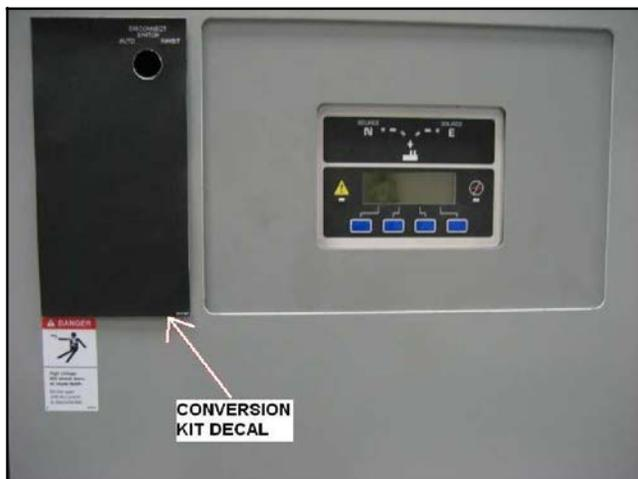
**Figure 32** Decal GM67498 Installed
