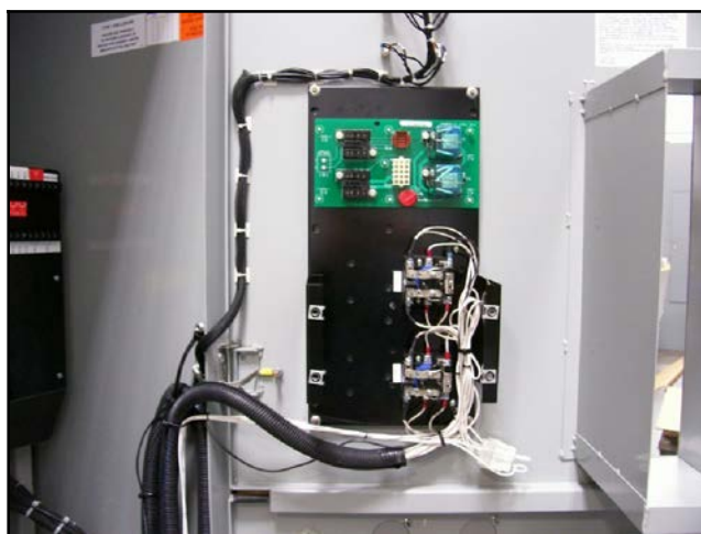
Figure 49 CCN and CCE Relay Location (see Figure 50 for other relays)
