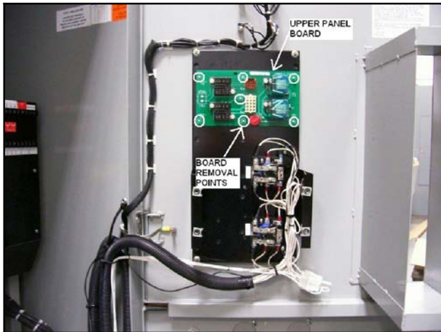
Figure 54 Remove the Upper Panel Circuit Board
