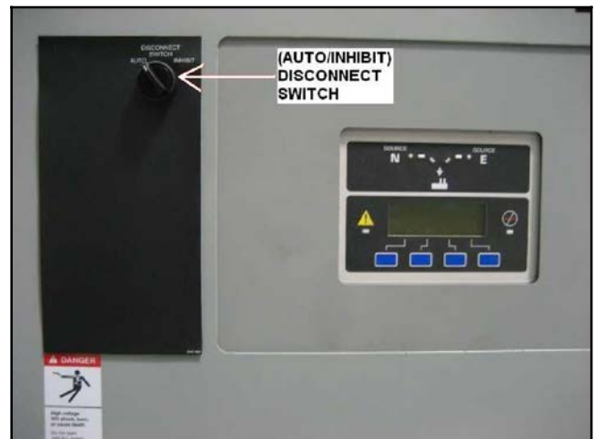
Figure 33 Disconnect Switch Re-Installed
