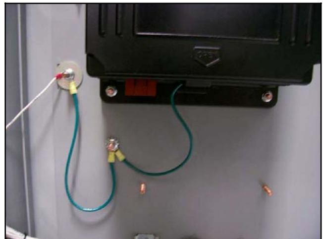
Figure 26 Ground Lead Connections
