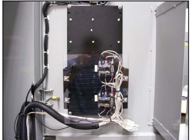
Figure 55 Re-Install Plastic Cover
