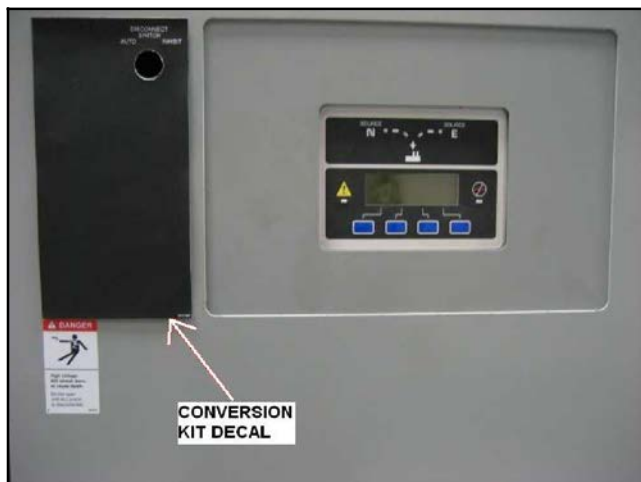
Figure 32 After Decal Installation
