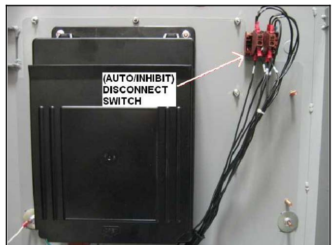
Figure 35 AUTO/INHIBIT Switch Connection
