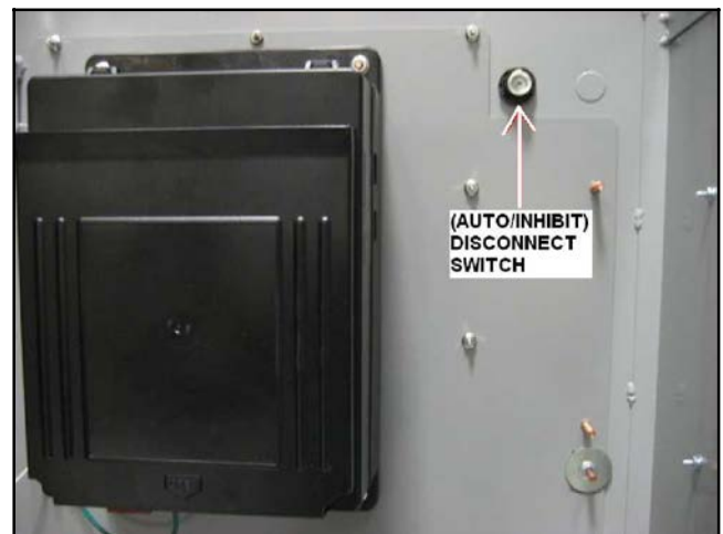
Figure 34 Disconnect Switch (inside door)
