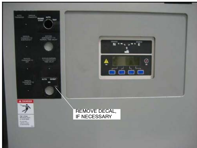
Figure 31 Before Decal Installation
