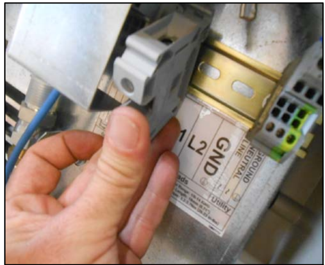
Figure 8 Installing the New Terminal Block
