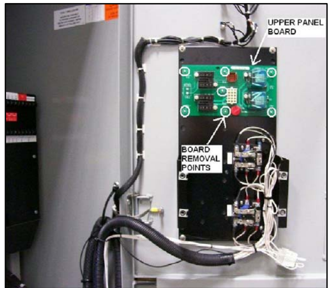
Figure 50 Remove the Upper Panel Circuit Board
