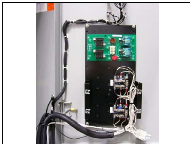
Figure 47 CCN and CCE Relay Location
