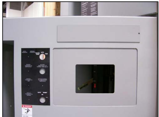
Figure 26 Door with Mounting Plate and Switch Cover Plate
