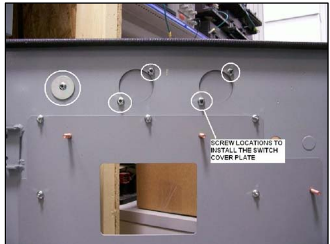
Figure 25 Switch Cover Plate GM69929
