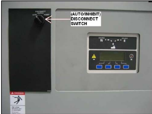
Figure 34 Disconnect Switch Re-Installed
