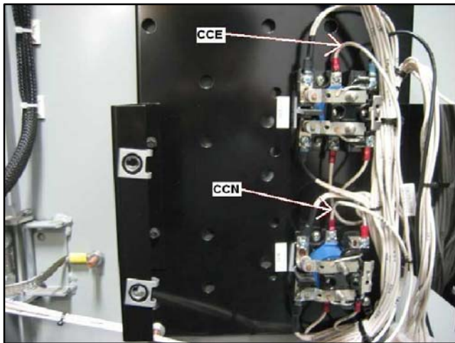
Figure 48 Connections to CCN and CCE Relays
