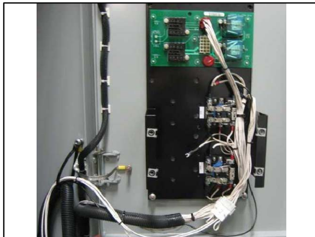
Figure 46 P8 has been disconnected from the upper board and connected to conversion kit harness GM69403.
