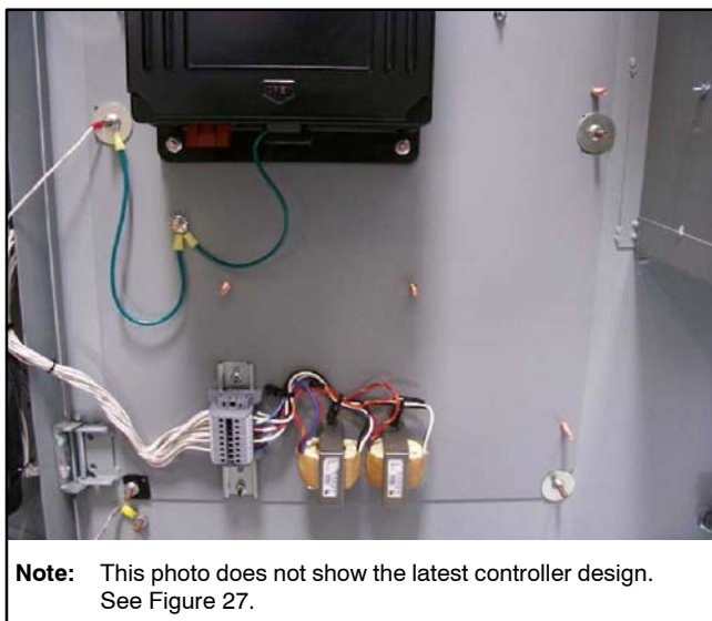
Figure 31 Transformers and Terminal Block Installed
