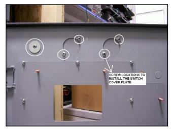
Figure 14 Switch Cover Plate GM69929
