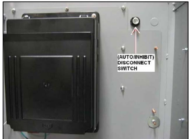
**Figure 33** Disconnect Switch (inside door)
