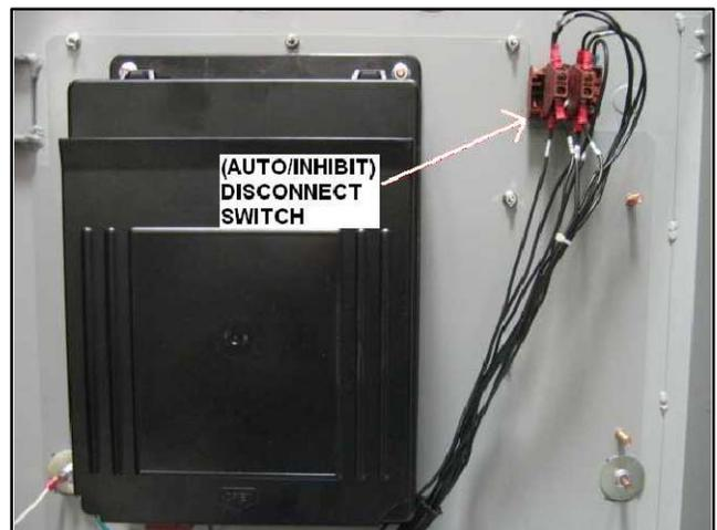
**Figure 34** AUTO/INHIBIT Switch Connection
