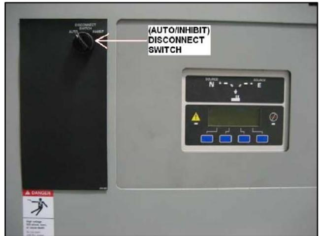
**Figure 32** Disconnect Switch Re-Installed
