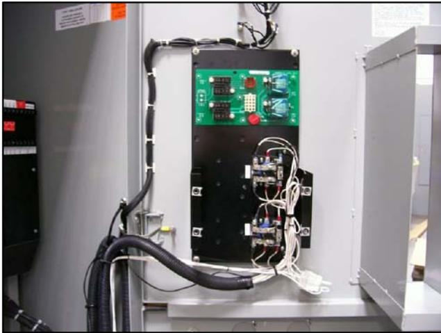
**Figure 48** CCN and CCE Relay Location (see Figure 49 for other relays)
