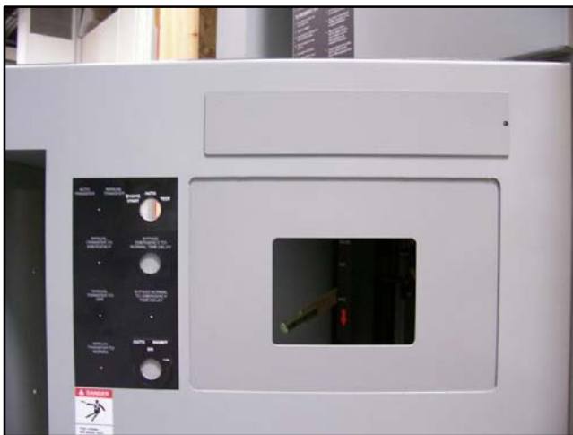
Figure 24 Door with Mounting Plate and Switch Cover Plate
