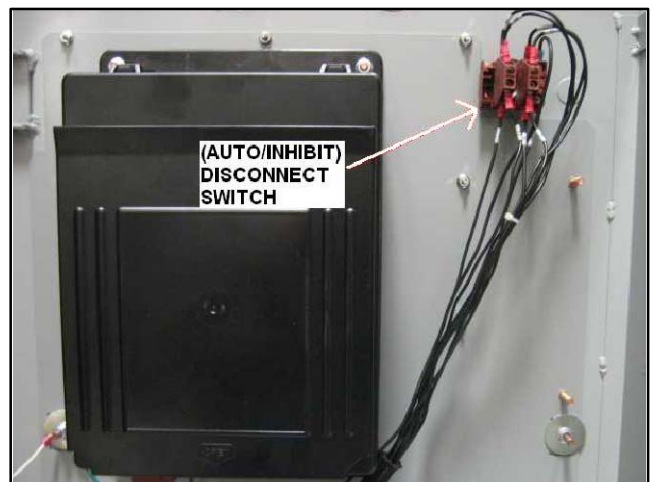
Figure 34 AUTO/INHIBIT Switch Connection
