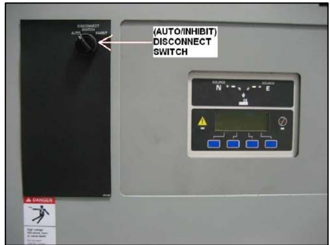
Figure 32 Disconnect Switch Re-Installed
