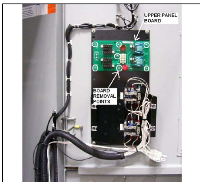
Figure 48 Remove the Upper Panel Circuit Board
