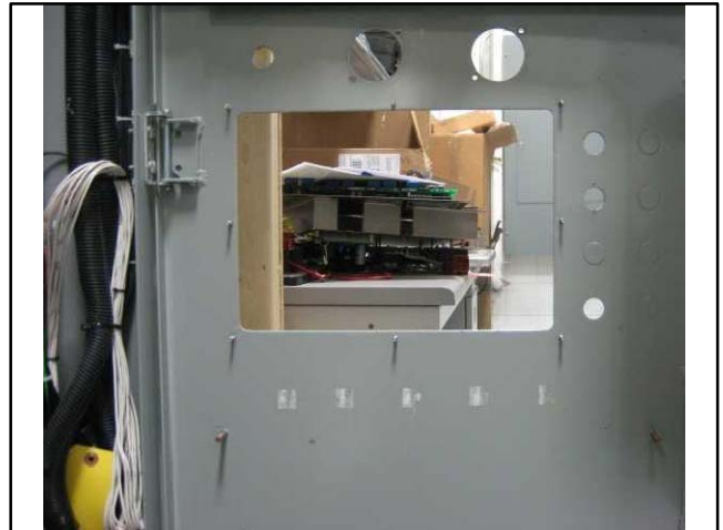
Figure 20 Controller and Lower Panel Removed
