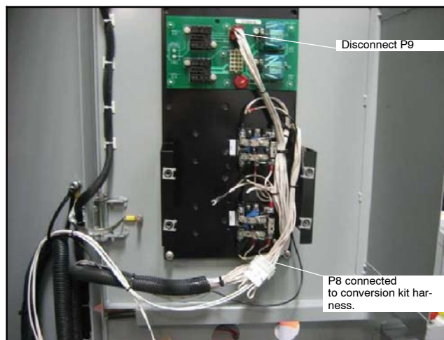
Figure 43 Disconnect P9
