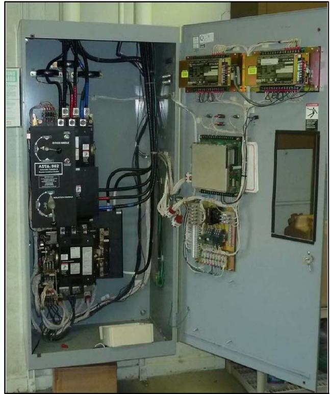
**Figure 6** Transfer Switch before Controller Replacement
