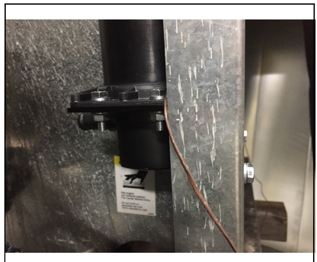
Figure 9 Location of Block Heater (Side view)
