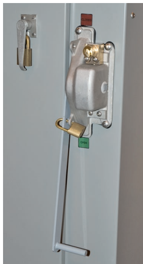
Figure 18. Key interlocks on manual switch-operating handle to guard against possible undesirable paralleling and to prevent opening the door unless downstream switches are open.
