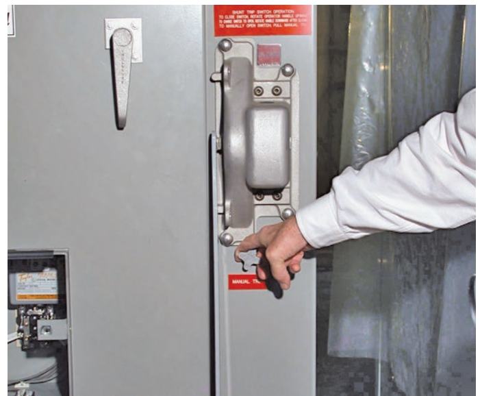
Figure 14. Manual Shunt-Trip Knob.
