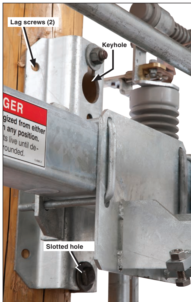
Figure 5. Typical mounting bracket attachment detail.
